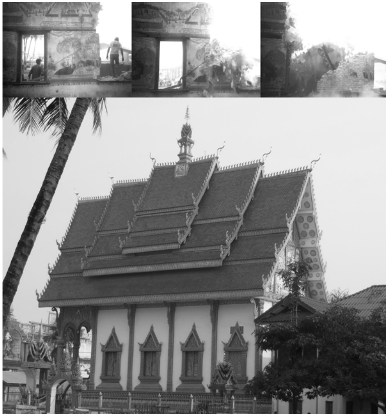
Figure 2. The old sim at Vat Ou Mong being demolished in December 2000 and the new sim completed.
